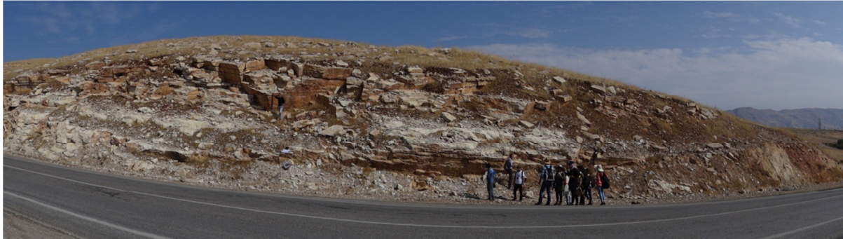
Fig. 6: Outcrops of the Turonian well bedded thick limestone Kometan Formation. The beds affected by highly fracture and faults. Location is the main road of Khalakan-Dokan main road, close to the Dokan Dam.
